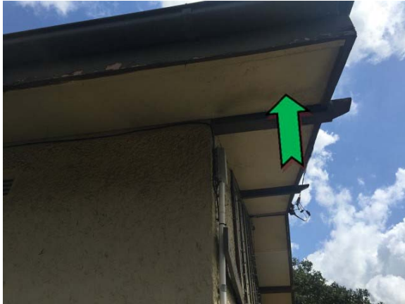
Photo 1. Exterior, throughout, eaves – non asbestos-containing fibre cement sheeting.
