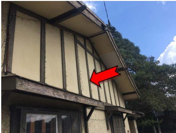
Photo 3. Exterior, east elevation, gable – asbestos-containing fibre cement sheeting.
