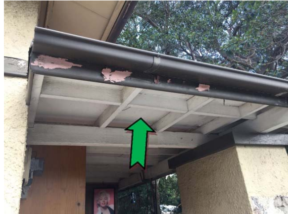
Photo 2. Exterior, north-east corner, awning – non asbestos-containing fibre cement sheeting.
